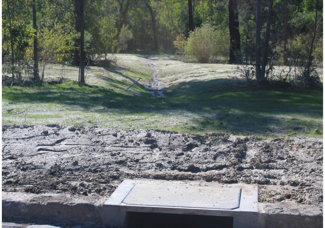
EnviroSeal is a process in which cellulose fibre, water and tackifiers are homogeneously mixed and sprayed to form a seal over areas where dust and erosion control are required. Tackifiers are sticking agents that bind soil particles together and protect the surface from wind and water erosion.
