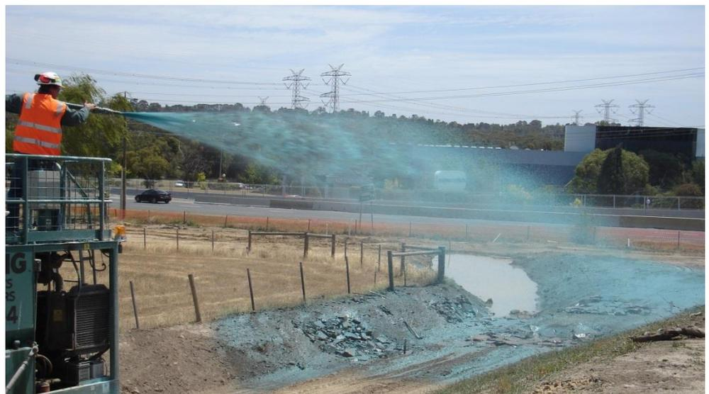
These spray-on technologies were developed specifically for large-scale applications on major earthworks projects where revegetation was a principal strategy for erosion control and where time and cost were critical. Rather than using built structures, such as masonry walls, natural vegetation is used for a "green" anti-erosion surface stabiliser.
